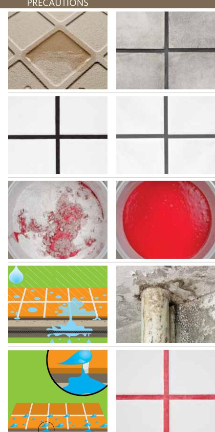
When components of the grouting material does not mix homogenously and with specified mixing rates, the final grout performance will fail, and therefore, the grout will easily be removed from its joint.
