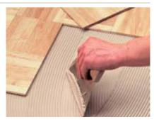
■ Adhesion and rigidity of the existing tile or PVC covering should be checked by tapping a hummer or scraper. Loose or poorly adhering covering should be removed and replaced by similar covering or the substrate should be reconstituted with a suitable repairing product.
